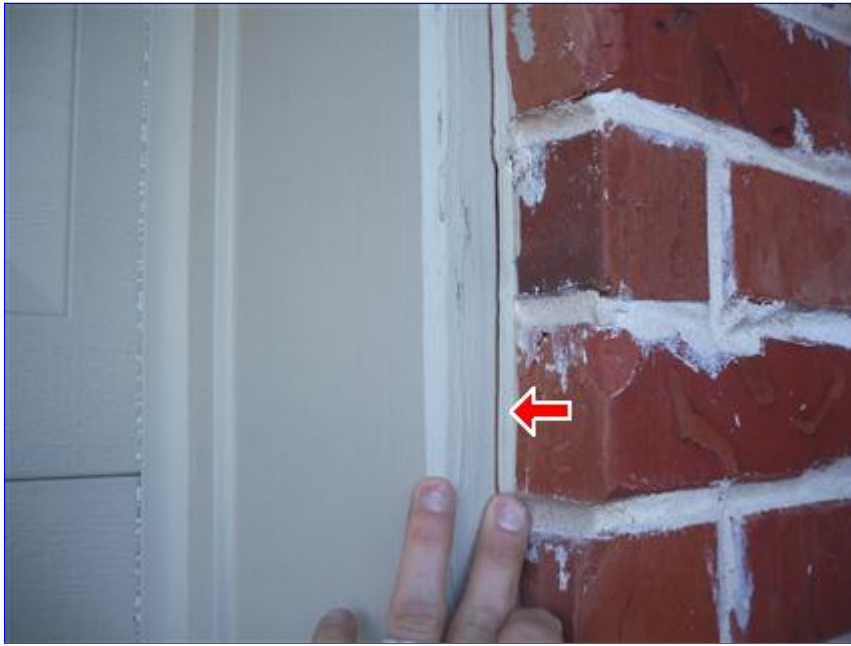
E. Picture 4 Garage
