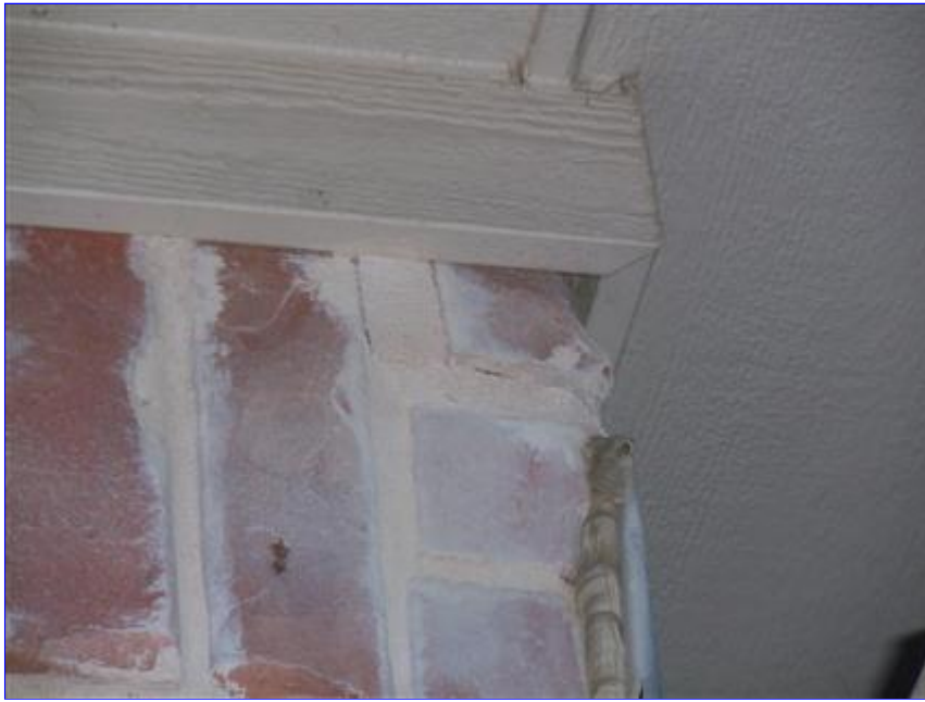
E. Picture 1 West side porch
